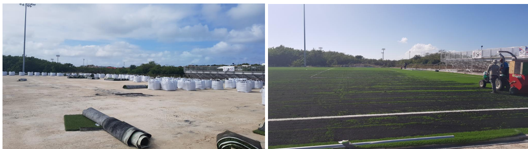
Repair, resurfacing, and replacement of the artificial turf
